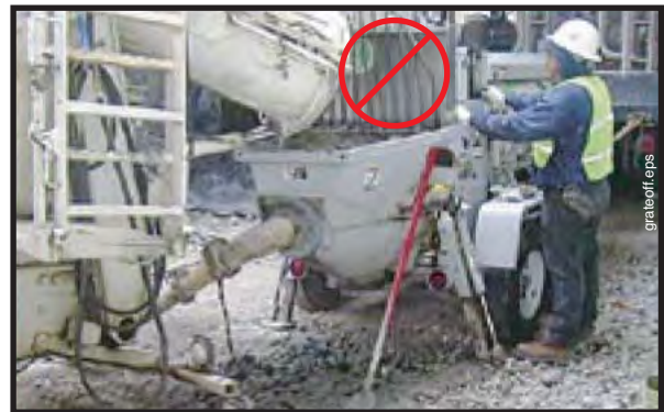
Figure 26 Never remove the hopper grate while the pump is operating
