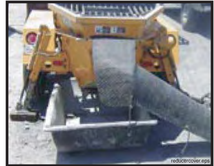
Figure 25 Cover reducers and use containment boxes for cleanout
