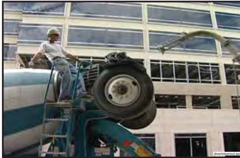
Figure 35 Divert vertical pipeline to the cleanout area and be sure to secure the discharge before continuing
